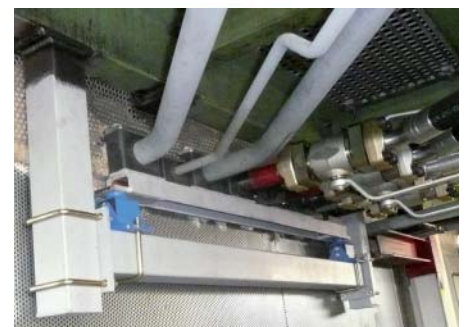
Yoke support installation
