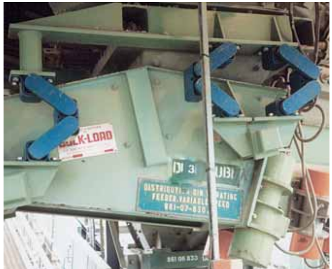
Hanging silo-discharge-feeder on AB
