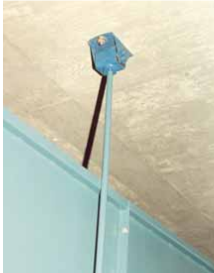
Belt conveyor hanging on type V
